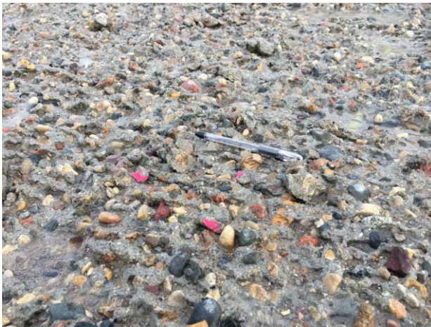
Figure 2-6. Substrate surface after hydro-demolition
