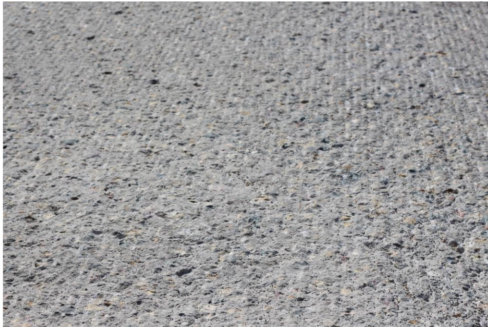
Figure 3-9. Photo of substrate surface condition of site E1
