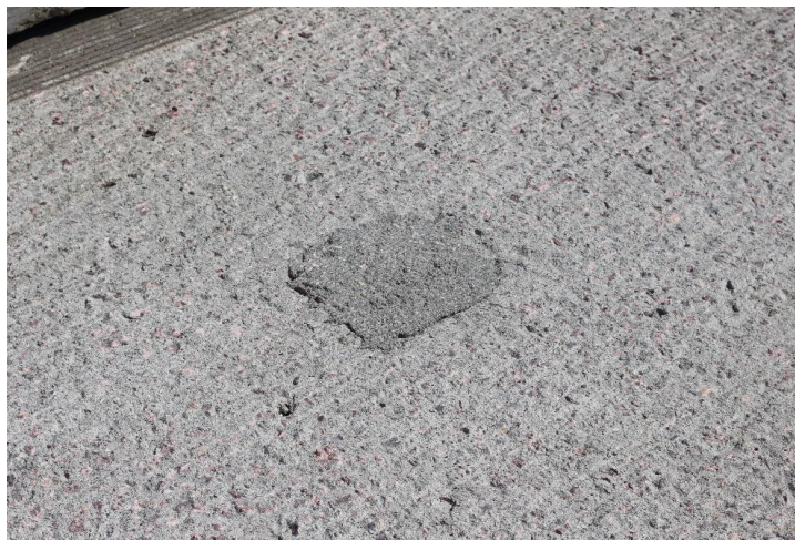
Figure 2-2. Repair of the substrate by patching
