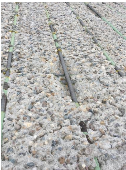
Figure 3-3. Photo of substrate surface conditions of site C1
