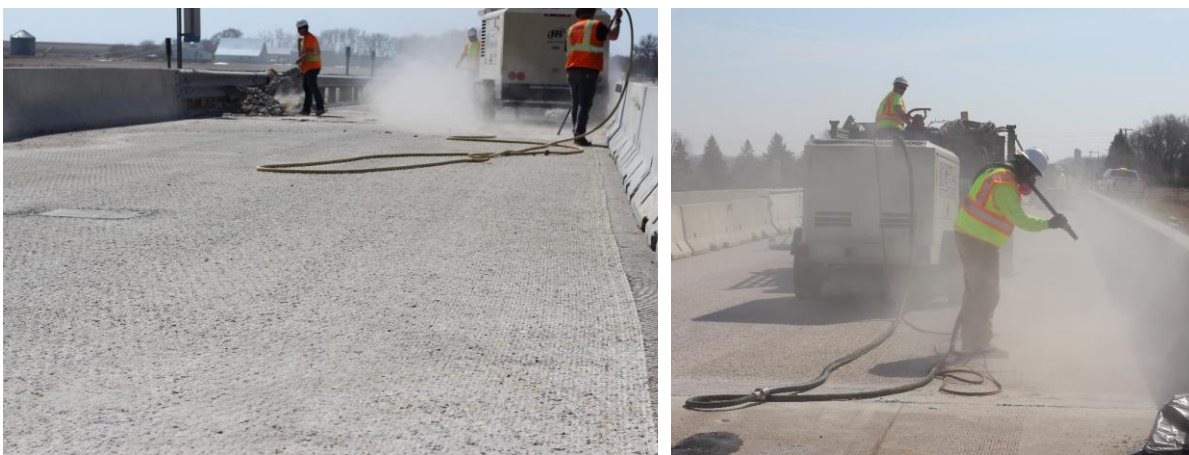
Figure 2-1. Cleaning the surface using compressed air (left) and sand blasting (right)
