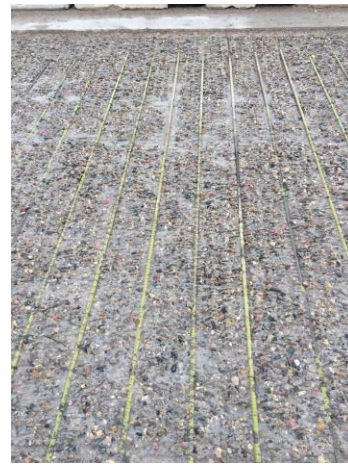
Figure 2-6. Substrate surface after hydro-demolition
