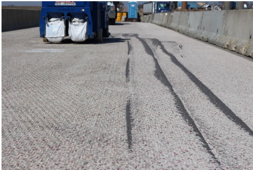
Figure 2-3. Shot blasting the substrate
