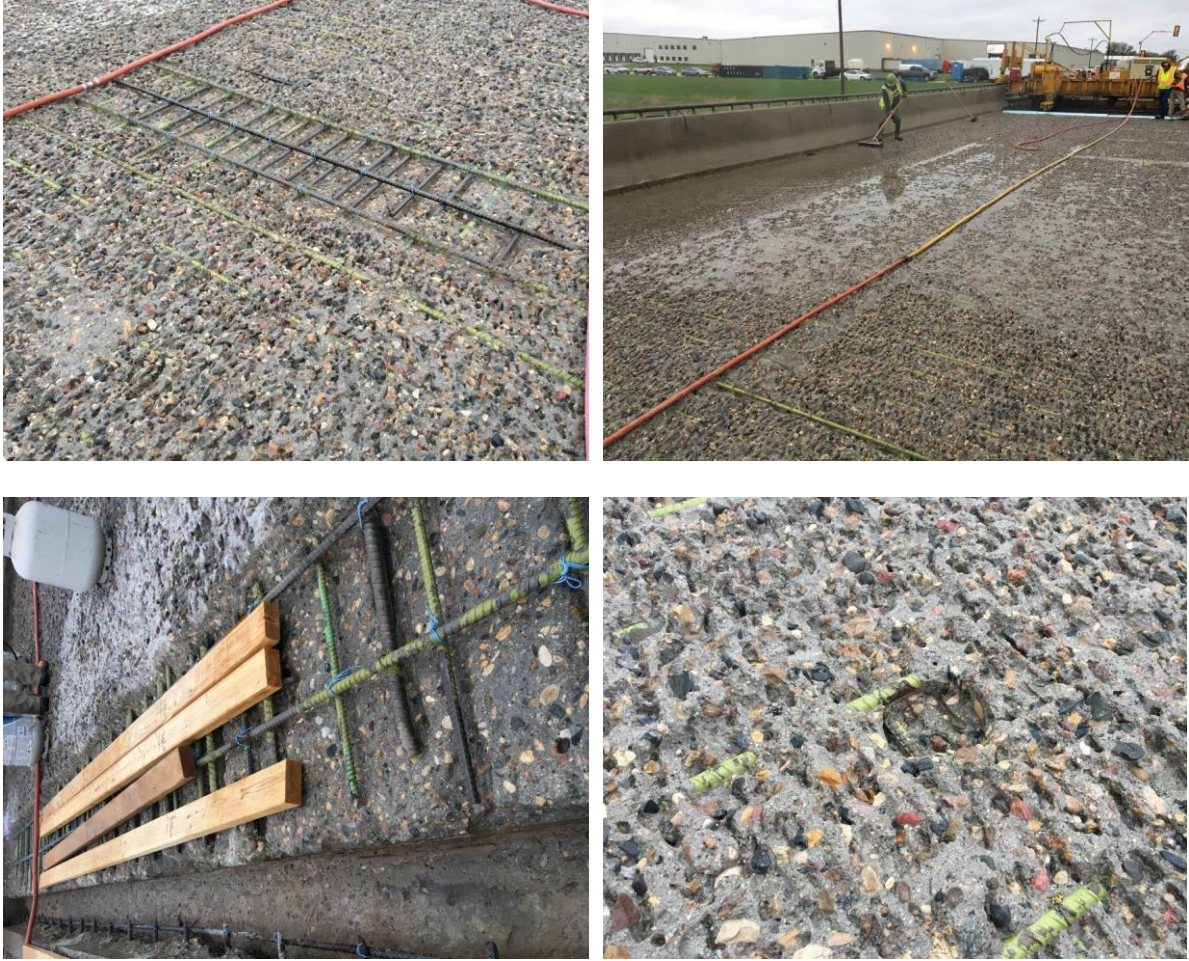
Figure 0-3. Surface condition of bridge deck of site C3 prior to overlay
