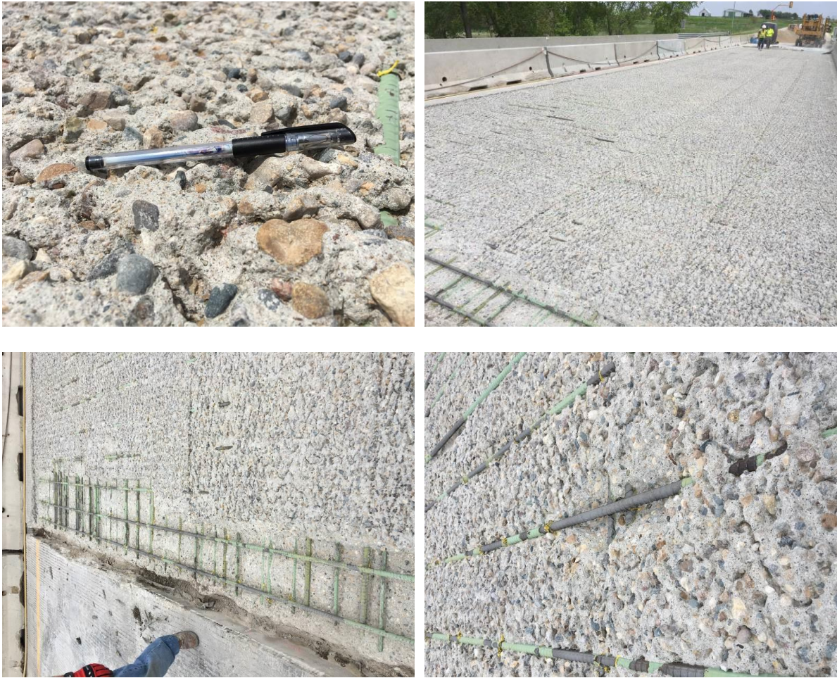
Figure 0-1. Surface condition of bridge deck of site C1 prior to overlay
